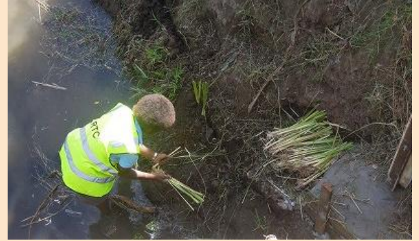
A woman plants native grass as part of a cash-for-work programme to protect the riverbank next to the market in Rakiraki.
